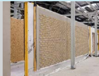
Brick slips applied to closed timber frame panel in factory manufacture.
