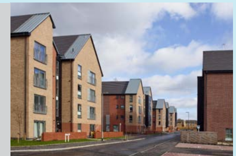
Closed panel system with brick slip facing as used in Queens Cross Housing Association development in Panmure Street, Glasgow.
