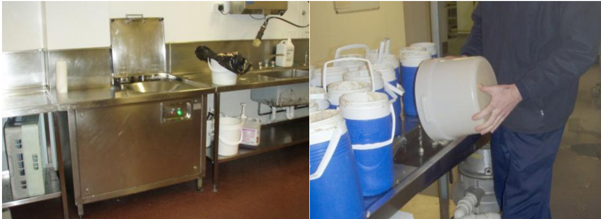
Figure 8: Vacuum and tank system, Ayrshire Central (left) and food waste bucket being emptied (right)
